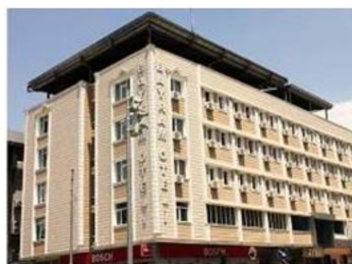
Fig. 2: Hotel Bayram of Van, before (down) and after (up) of its collapse in the aftershock of 9 November 2011, M5.6 (3, 4)
